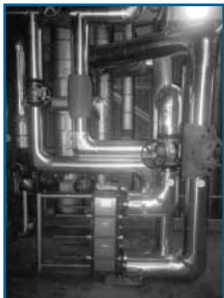
Augusta Newsprint installed a plate-style, boiler blowdown to preheat boiler make-up water.
